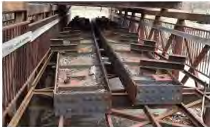
Condition of Talbot Avenue Bridge plate girders (March 22, 2023)
