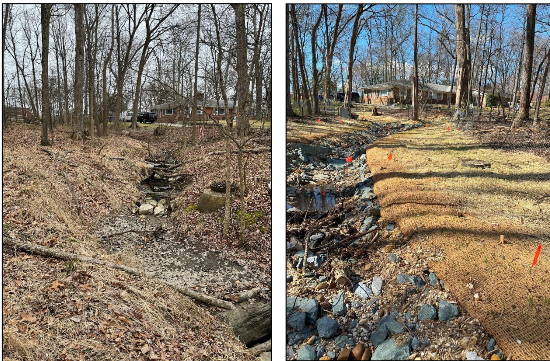
Above: Parker Avenue outfall restoration facing upstream (left is prior to construction and right is immediately following construction; the sewer manhole is visible in both photos).
