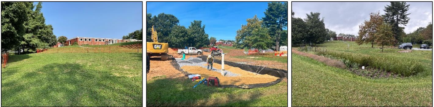
Figure 3. Installation of a micro-bioretention at Colesville Local Park to treat previously untreated stormwater runoff from the parking lot
