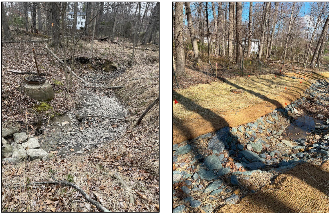
Above: Parker Avenue outfall restoration (left is prior to construction and right is immediately following construction; the sewer manhole on the left bank is visible in both photos).
