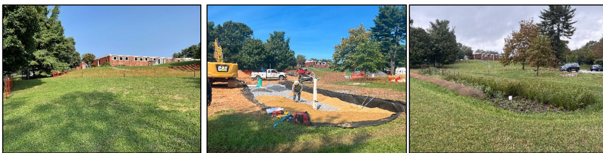
Above: Colesville LP Micro-bioretention before, during and after construction.
