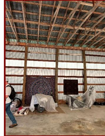
View of west side of structure. Note hurricane ties connecting trusses to spandrel beams.
