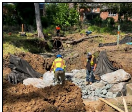
Byeforde Road outfall during construction
