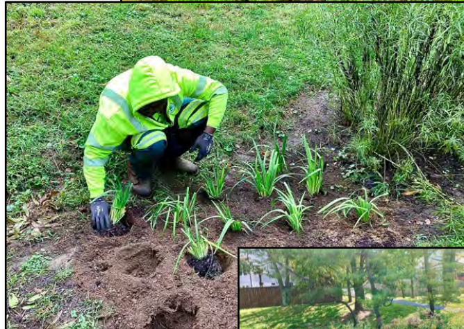
Montgomery Parks staff plant native species in a stormwater bioretention facility
