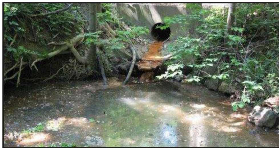
Orange flocculant accumulating in an outfall. Photo by Geoffrey Mason.
