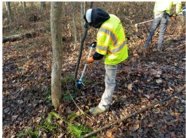
Pictured above (left) is the dauber tool. The sponge tip is on the left and the control valve on the right. Right, is a pesticide applicator carefully applying product to a cut stump. The adjacent ferns are protected from this application by the dauber tool.
